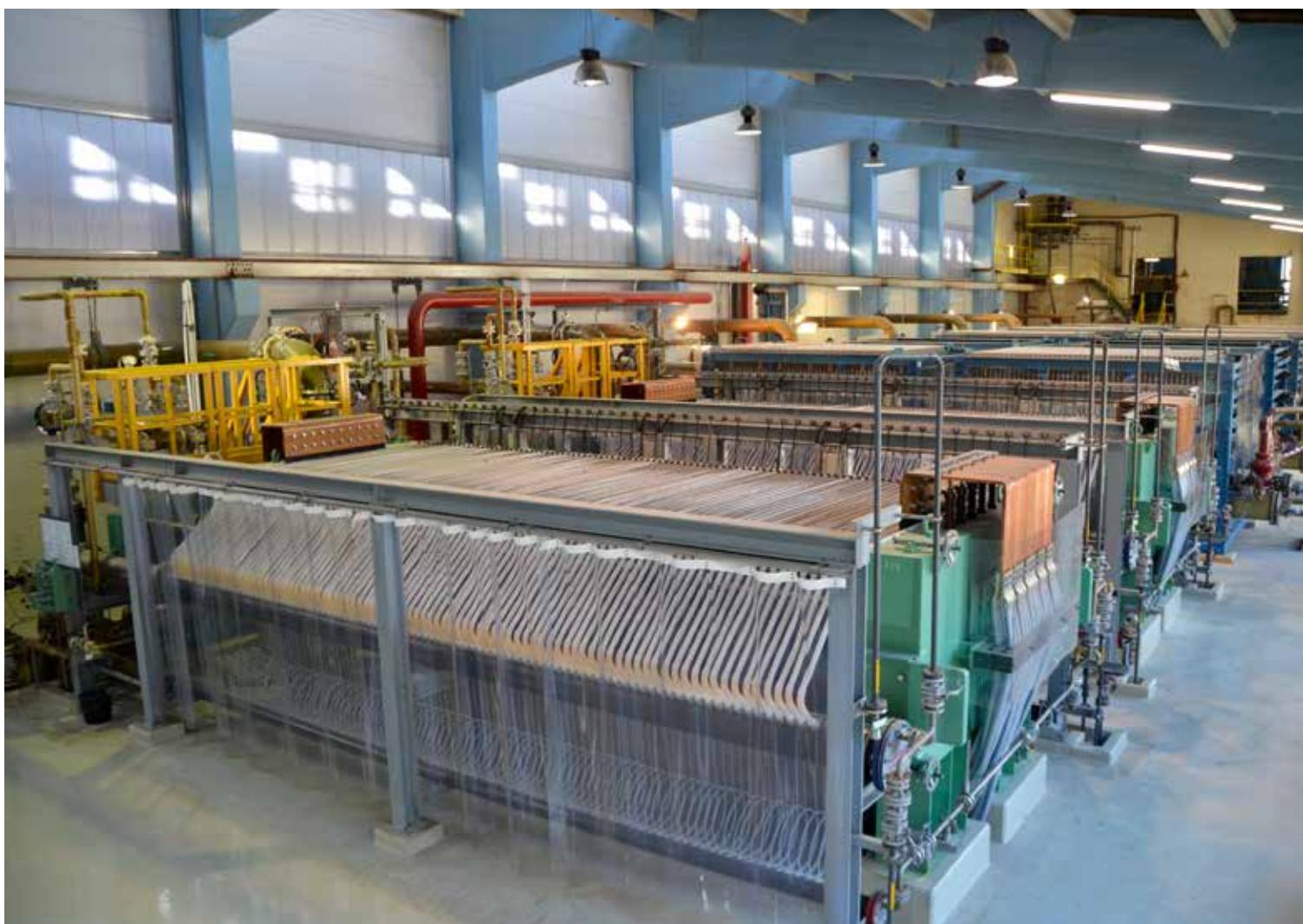
With zero-gap technology energy requirements are reduced by around ten percent.
