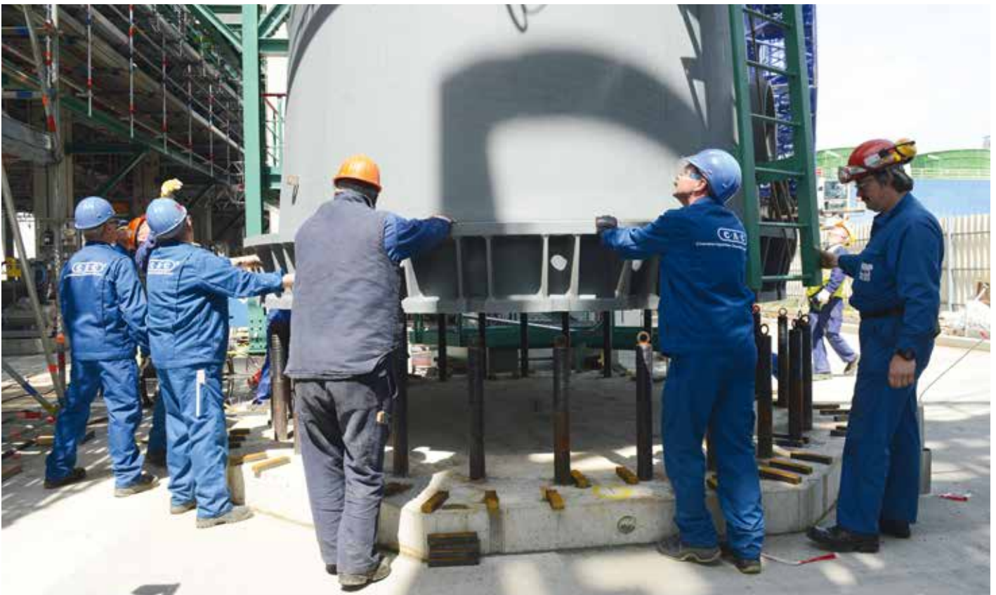
Alignment of the columns has to be undertaken by hand.
